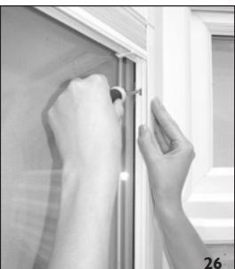
Remove one side at a time to ensure easier removal (Fig. 27).
